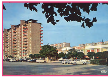
Reconstruction, Sotteville-les-Rouen. Grand ensemble Zone verte. 1050 logts.
